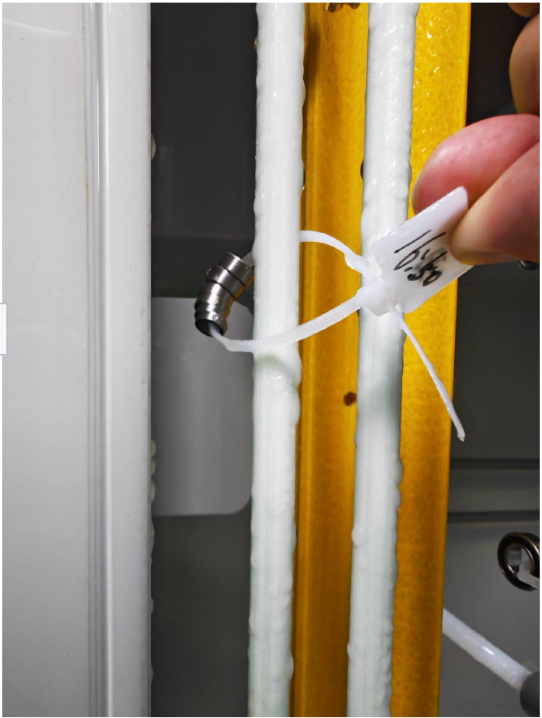
Close-up after exposure — no corrosion
